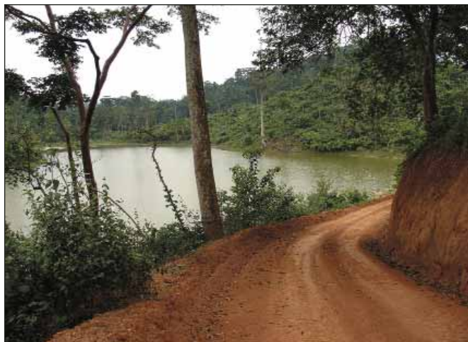
Chirano Water Storage Facility
