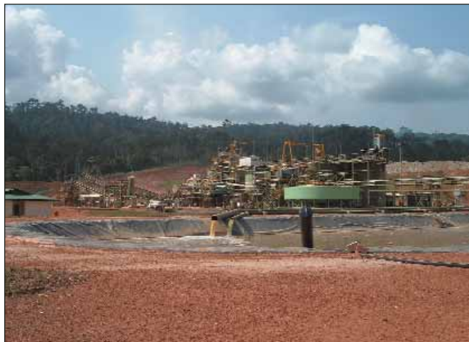
Chirano Process Plant
